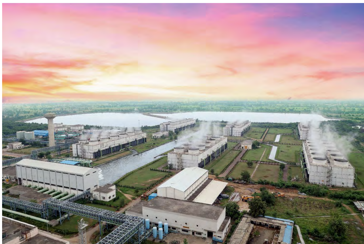
Lalitpur Power Plant
