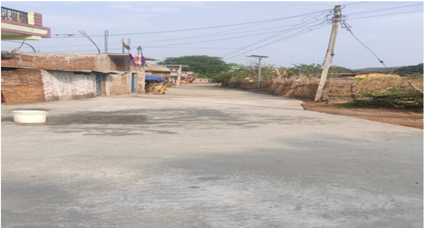
PCC Road constructed at Poraiya village: CSR, Tilaiya Dam
