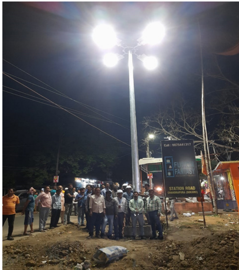
Installation of High Mast Light by CSR Chandrapura TPS
