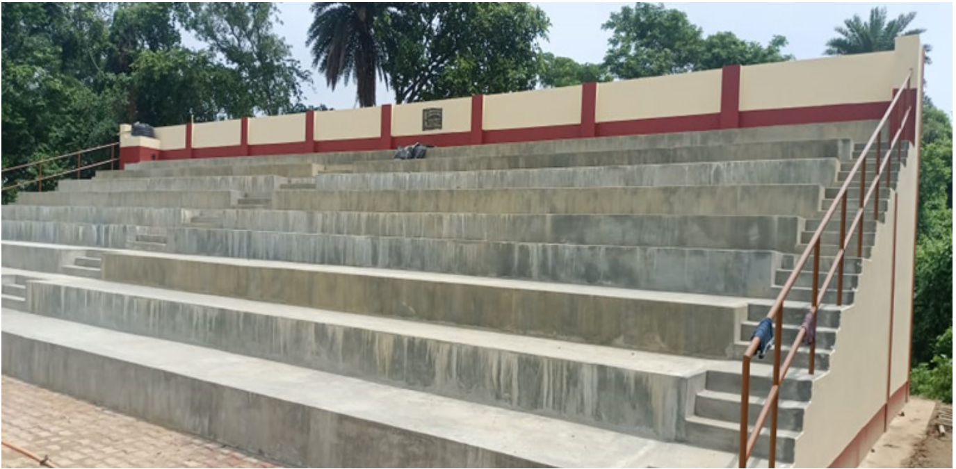
Gallery at Madanpur Football Ground constructed: CSR, Durgapur Steel TPS
