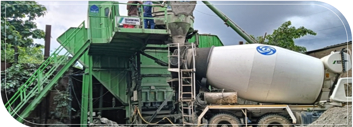
BATCHING PLANT WITH TRANSIT MIXTURE
