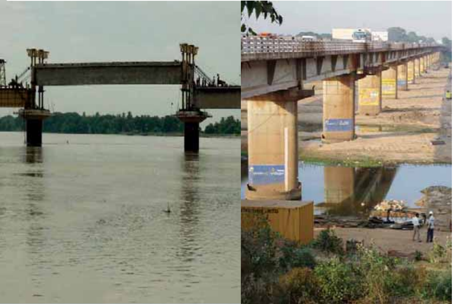
Precast Prestressed Girder of 43.5m span being erected for Railway Bridge on Luna River in Orissa for M/S RVNL
