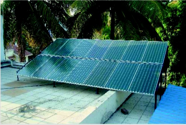
Pune, 1KWp rooftop system for a residence
