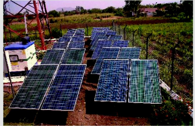
Solar powered telecom tower with total capacity of 6KWp
