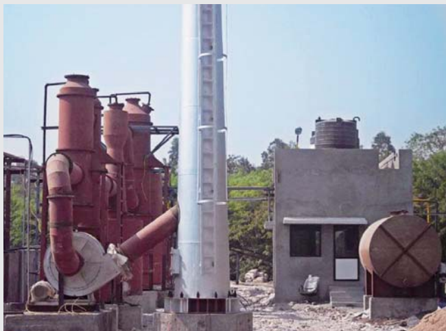
Captive incinerator for organic waste at Bhestan
