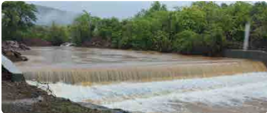
➤ A serene glimpse of the water reservoir after renovated under holistic village development project now flowing steadily
