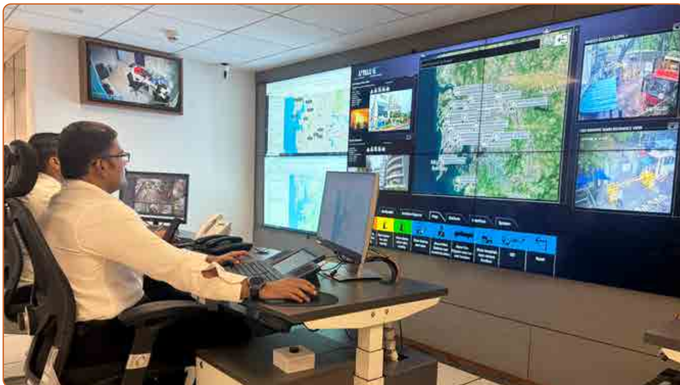
Integrated Security Control Room at MGL Mahape Office
