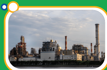
Primary & secondary structures for boilers & turbine generators
