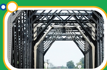
Railway's, Roads, bridges & girders
