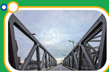
Structures for roads & bridges
