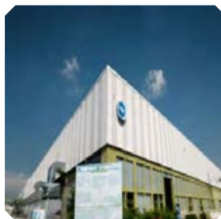
Corporate offices, information technology (IT) parks, industrial complexes
