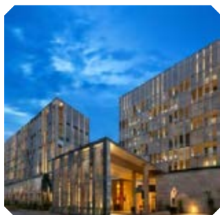
Hotels, institutional and hospital buildings
