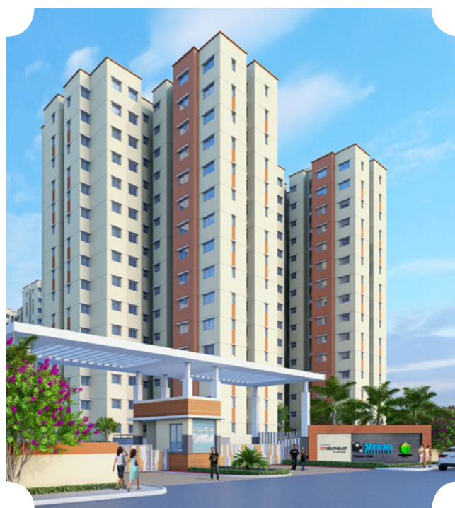
↑ Shriram 107 South East
