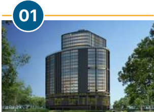
0.9 msf at CIGNUS POWAI® Tower II
