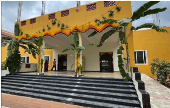
Construction of a Dormitory Building for Residential Students at Vishwakshema Trust
