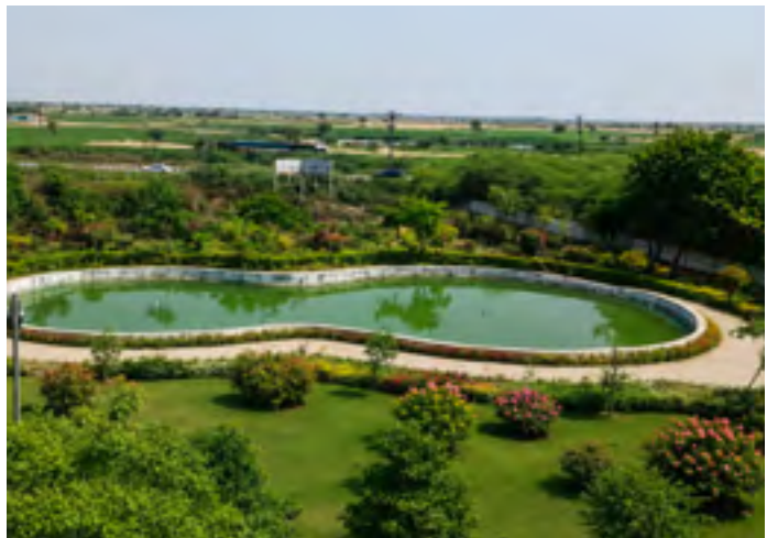
Water Conservation at Sanand Plant
