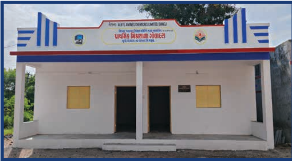
Construction of two class rooms at ZP School, Goladara – Dahej, Gujarat
