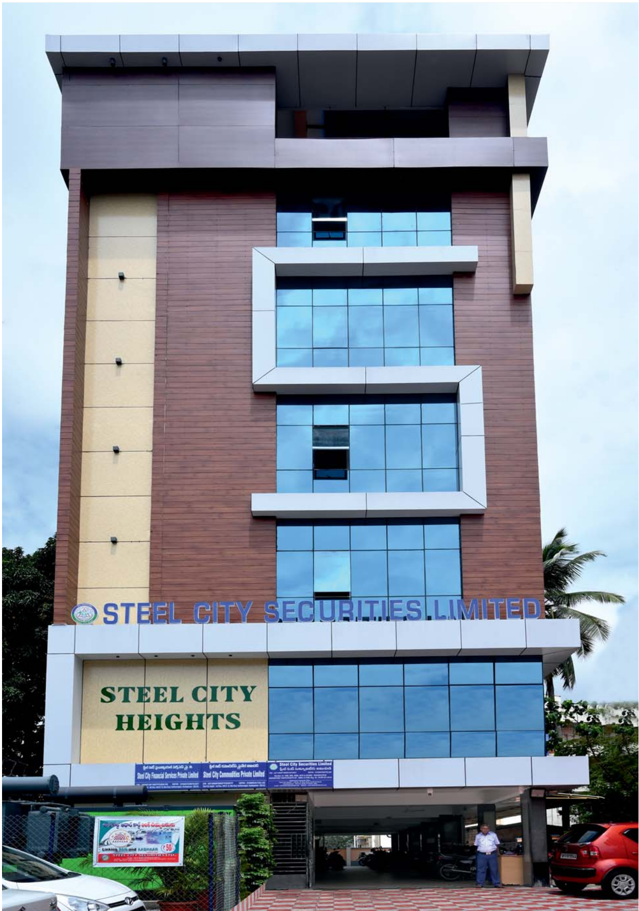
REGISTERED AND CORPORATE OFFICE BUILDING
