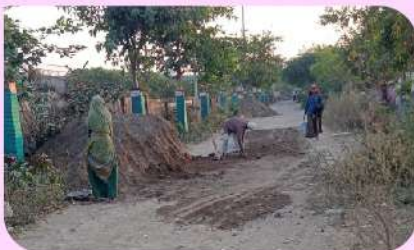
Road Renovation Projects.
