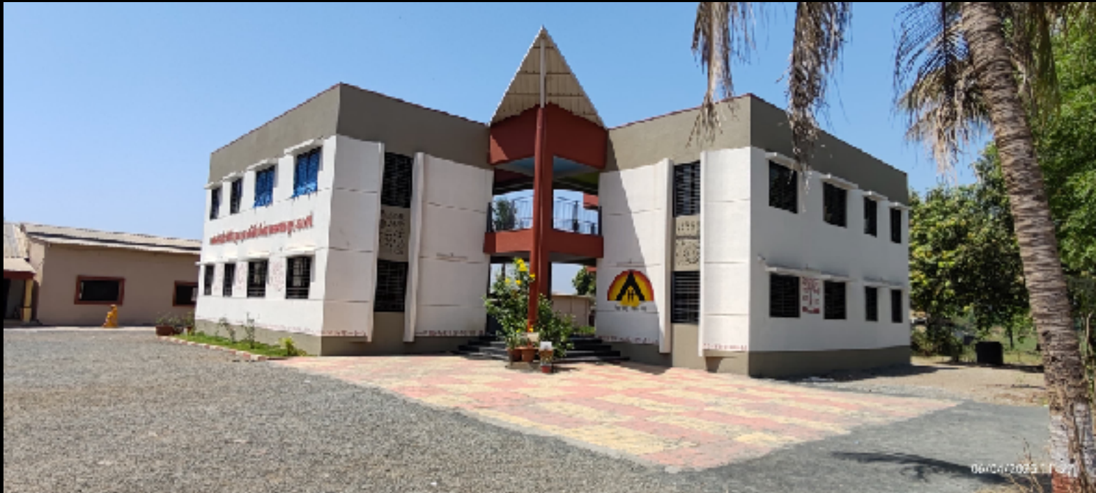
Constructed Vinoba Ashram Shala, Gadat, Gujarat | 20.9816158 ° N | 73.3544573 ° E
