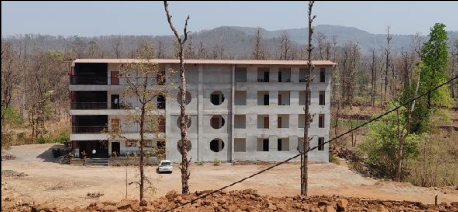
Under construction, S S Mahla School, Dang, Gujarat , for women empowerment | 20.8025303 ° N | 73.5392216 ° E
