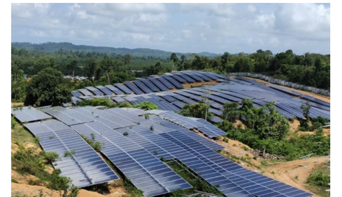
20 MW plant in Port Blair, Andaman and Nicobar Islands
