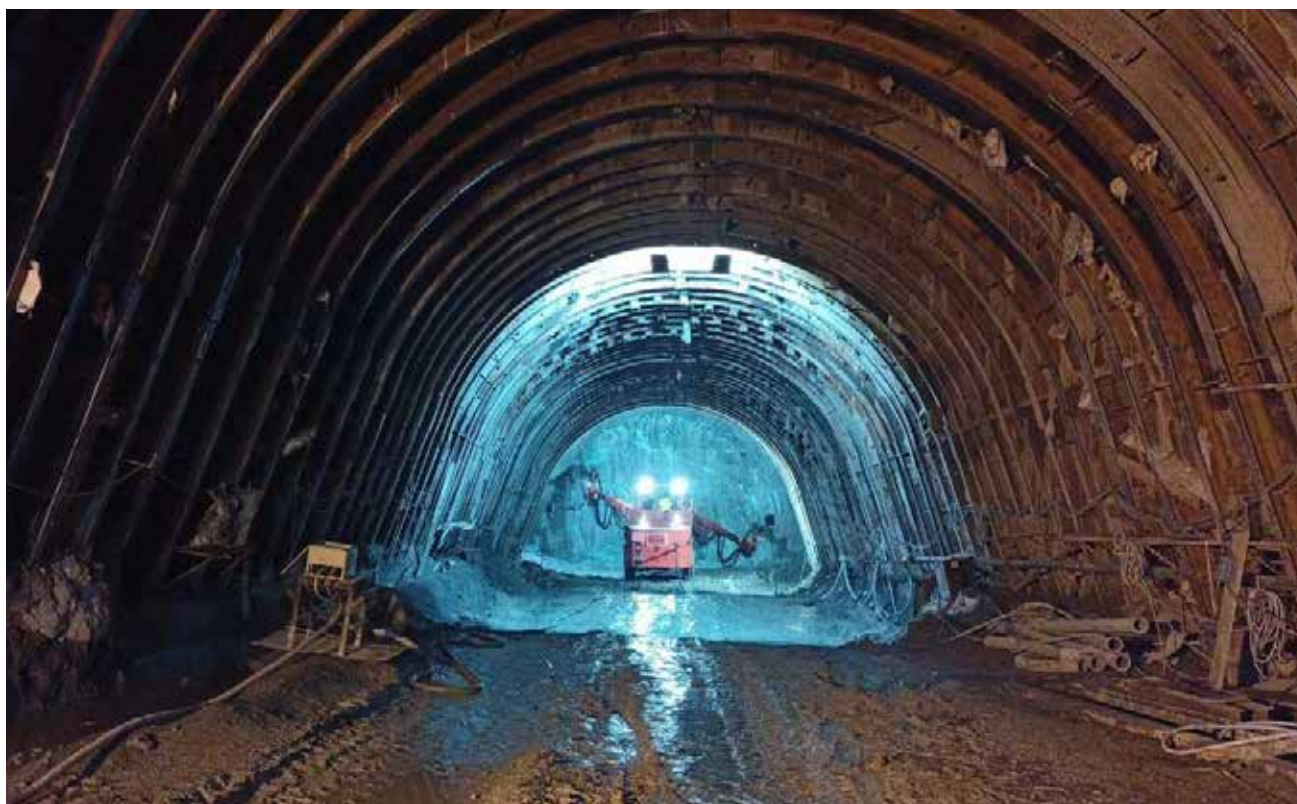
HEADING EXCAVATION OF MAIN ACCESS TUNNEL #1 - 2880 MW DIBANG MULTIPURPOSE PROJECT (ARUNACHAL PRADESH)
