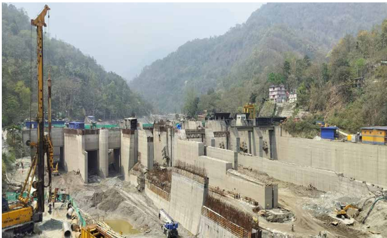
26.5 M HIGH BARRAGE UNDER CONSTRUCTION – 500 MW TEESTA-VI (SIKKIM)
