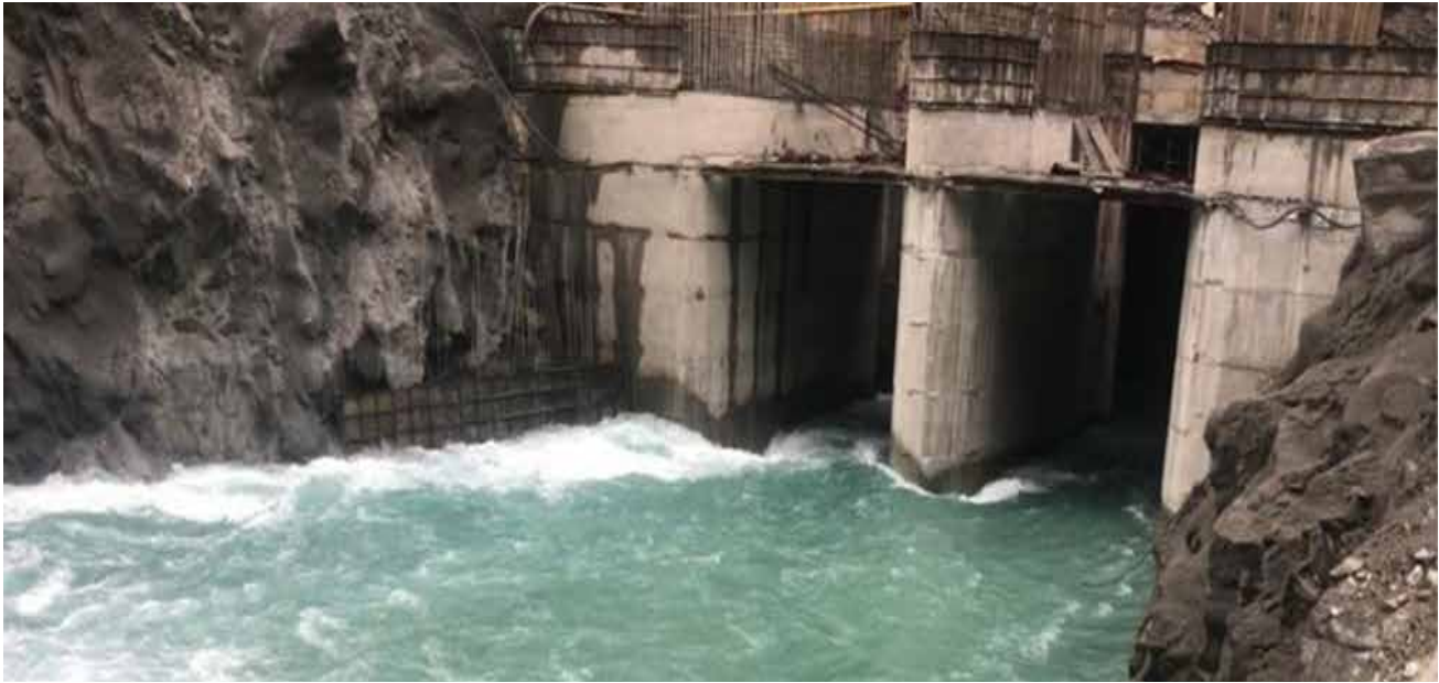
RIVER DIVERSION ACHIEVED ON 15.01.2024 – 540 MW KWAR (UT OF J&K)
