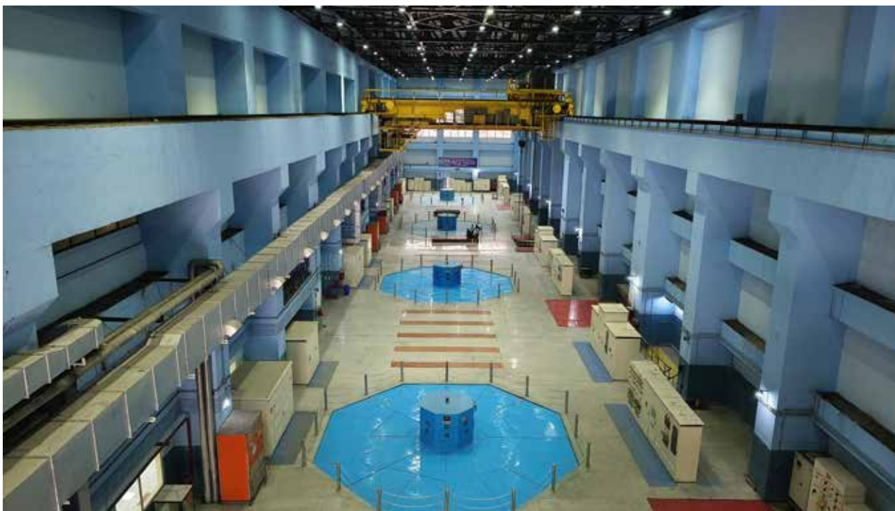
SURFACE POWER HOUSE– 800 MW PARBATI-II (HIMACHAL PRADESH)
