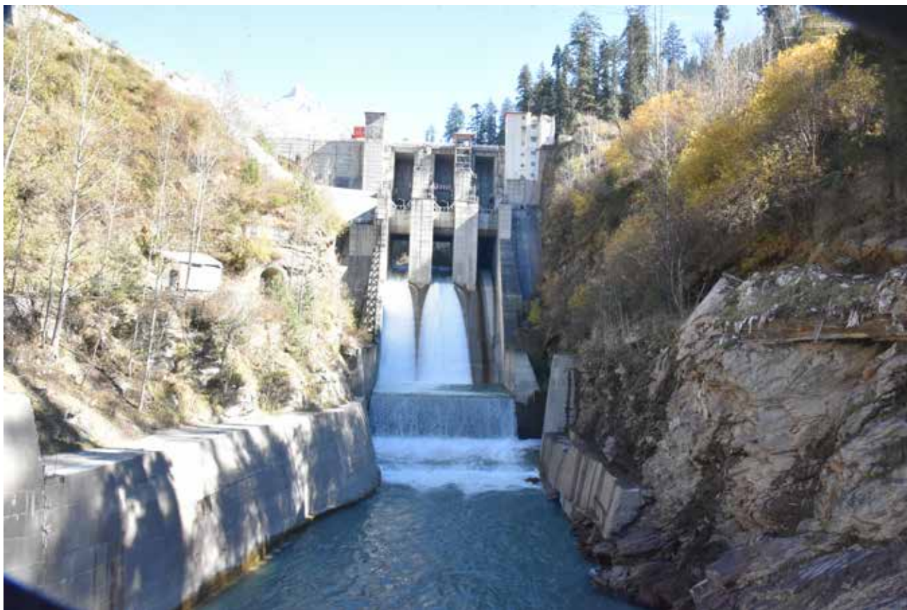
83.7 M HIGH CONCRETE GRAVITY DAM – 800 MW PARBATI-II (HIMACHAL PRADESH)
