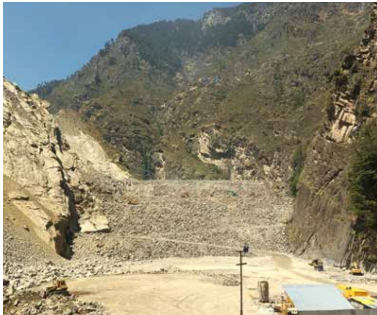
FILLING OF 167 M HIGH CONCRETE FACE ROCK FILL DAM – 1000 MW PAKALDUL (UT OF J&K)
