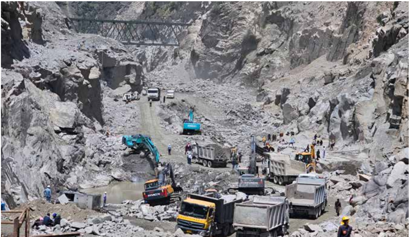
DAM PIT EXCAVATION – 540 MW KWAR (UT OF J&K)
