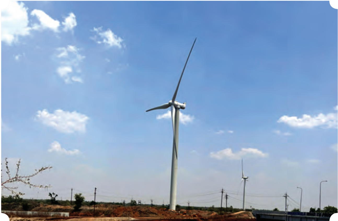
20MW Wind Energy project in Nipaniya, Mandasaur, Madhya Pradesh financed by REC
