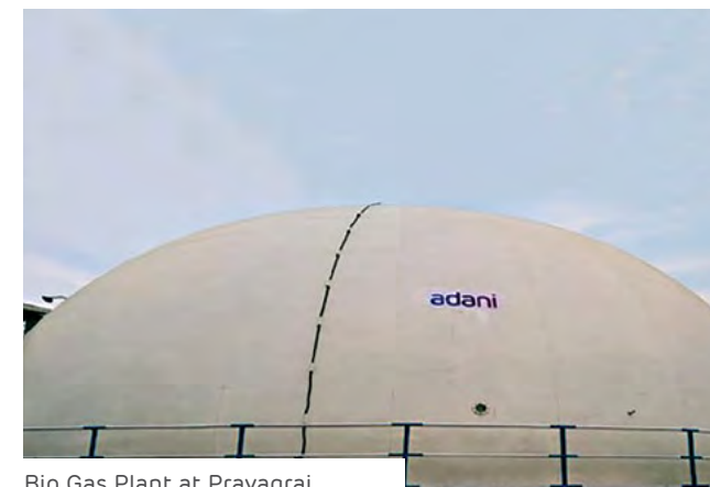
Bio Gas Plant at Prayagraj
