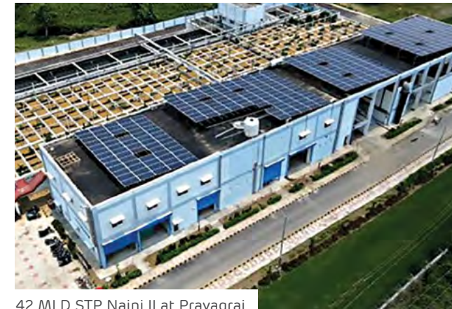
42 MLD STP Naini II at Prayagraj
