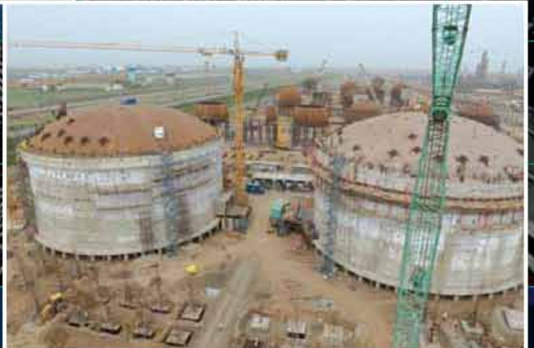
Double Walled Pre-stressed Cryogenic Tank at Dahej, Gujarat
