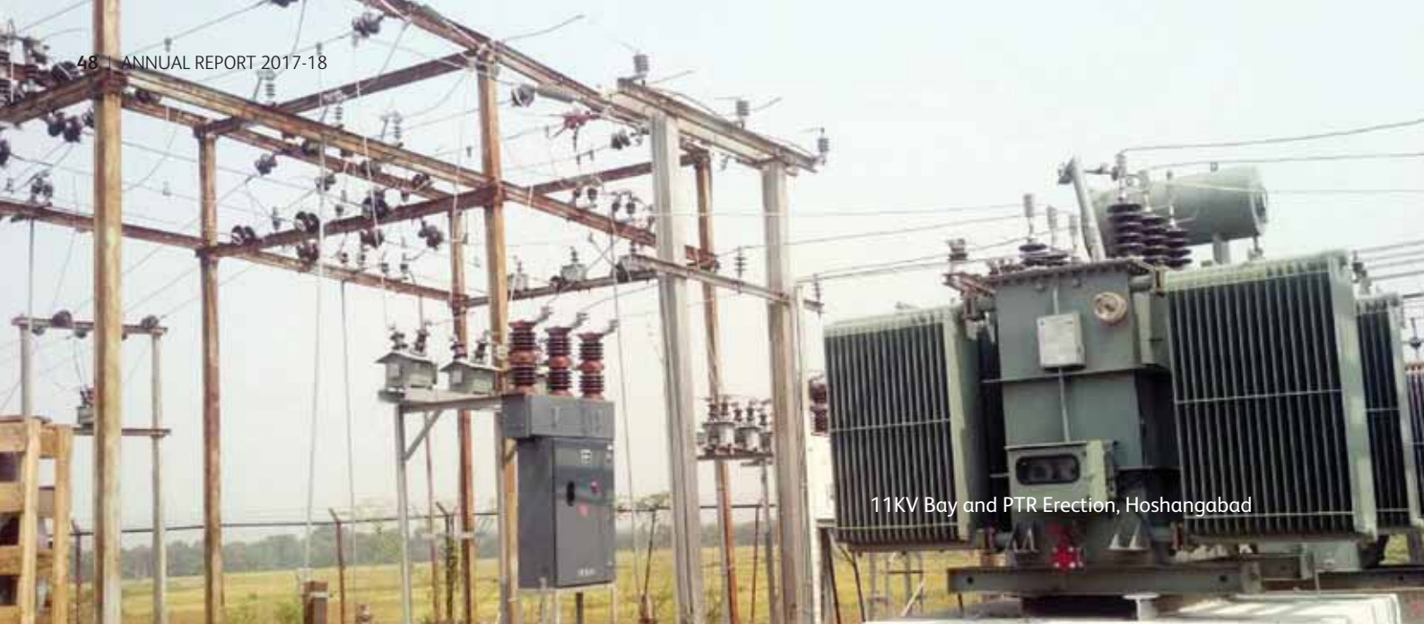
Erection of 33/11 KVA, 5 MA Power transformer, Hoshangabad
