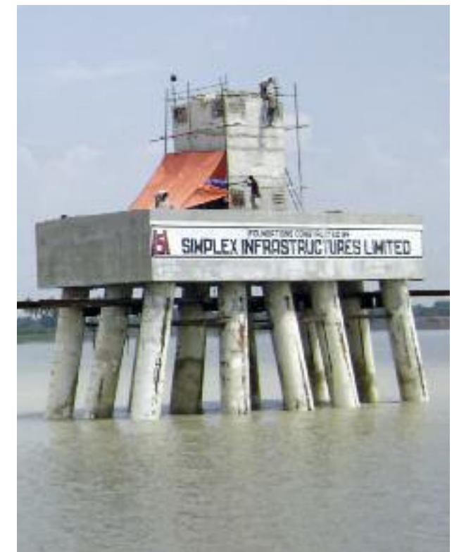
Raked Steel Pile & Cap Foundation for 240M High Transmission Tower for 400KV DC Line across Hooghly River at Raichak to evacuate Power from CESC's Haldia unit to Kolkata
