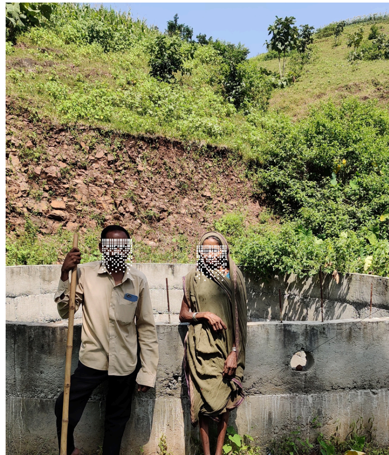
NEWLY CONSTRUCTED WELL FOR IRRIGATION, 5 FARMERS USING THE WATER FOR VEGETABLE CULTIVATION
